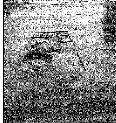
Figure 4: Both patches improperly backfilled and compacted and not patched to the nearest joint of seam.
